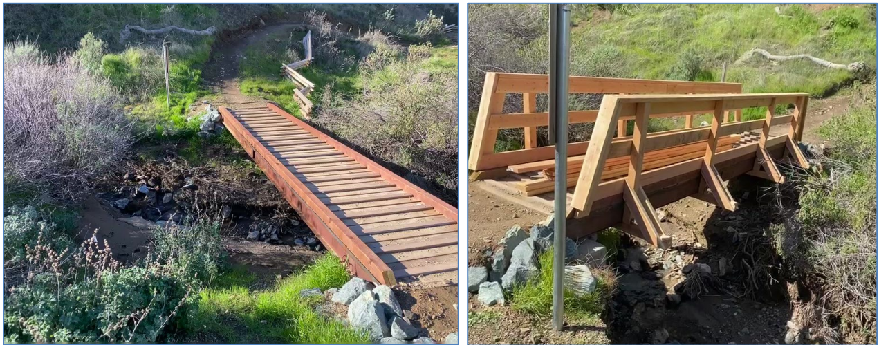
Figure 2-23: Bunkhouse Bridge without Railing (Left) and with Railing (Right)
